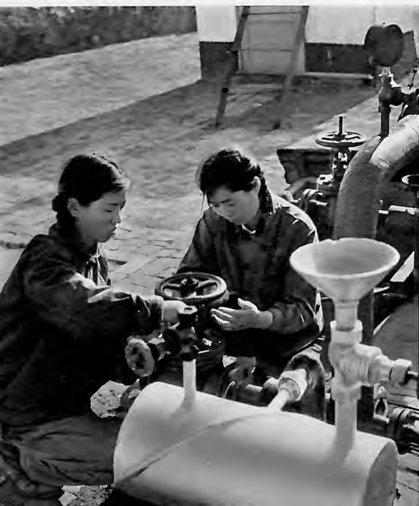
Checking and repairing an oil-well installation.
